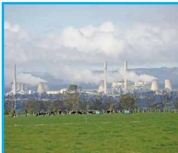
A coal power station in Victoria. The combustion of carbon produces considerable heat to produce steam to turn turbines to produce electricity. \text{C} + \text{O}_2 \rightarrow \text{CO}_2 + \text{heat}
