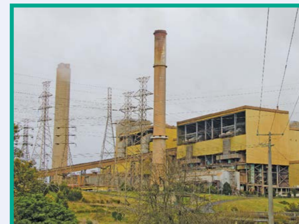
A coal power station in Victoria. The combustion of carbon produces considerable heat to produce steam to turn turbines to produce electricity. \text{C} + \text{O}_2 \rightarrow \text{CO}_2 + \text{heat}
